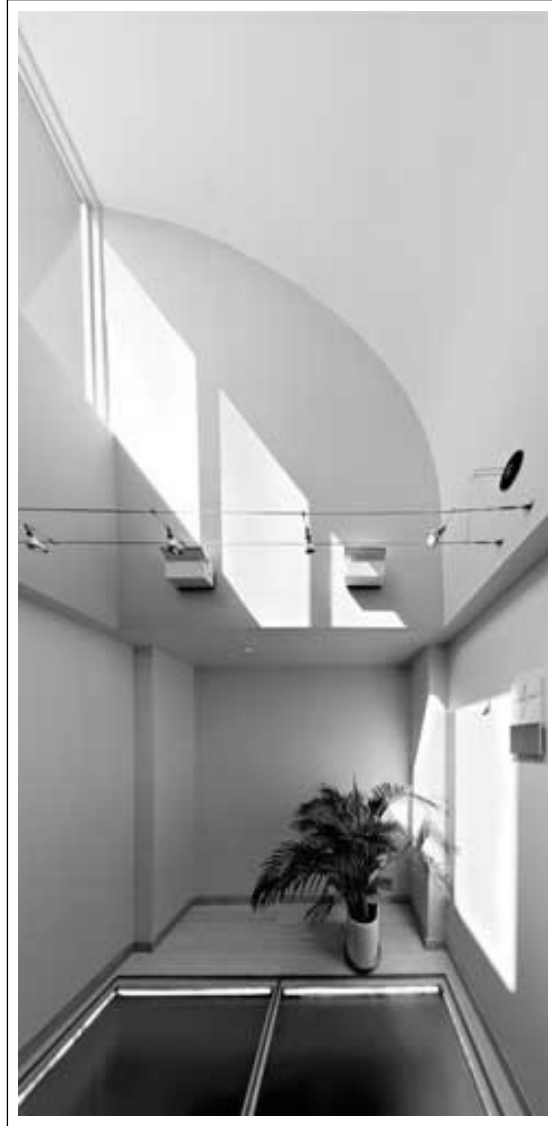
Figure 6. FCNL Building, interior with light scoop
