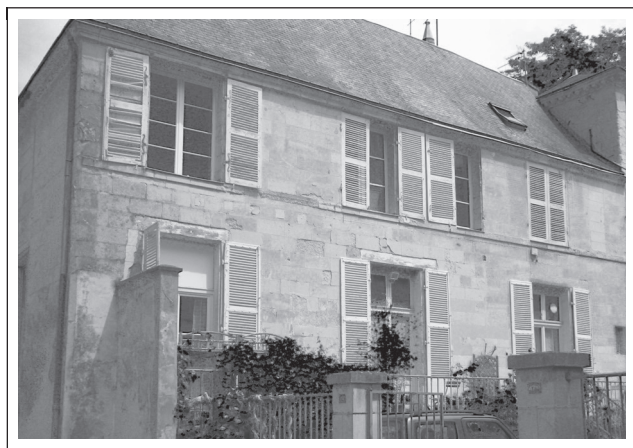
Figure 7. House believed to have been a boarding house for students at the Protestant Academy.
